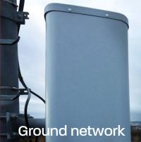
The ground network consists of A2G base stations, which get installed on existing towers of our Mobile Operator partners. These base stations are built upon open-standard 4G and 5G components and configured with special antennas, which create a dense network of cells in the sky that provides its maximum throughput to each aircraft.
